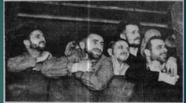
Workers inside Fisher Body 1
